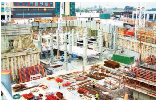
Basement Construction; showing the triple height columns & precast retaining walls
